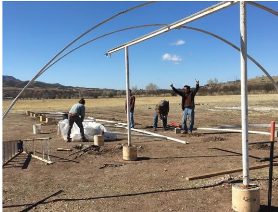
Greenhouse construction in action! [p.c.- BRN]
